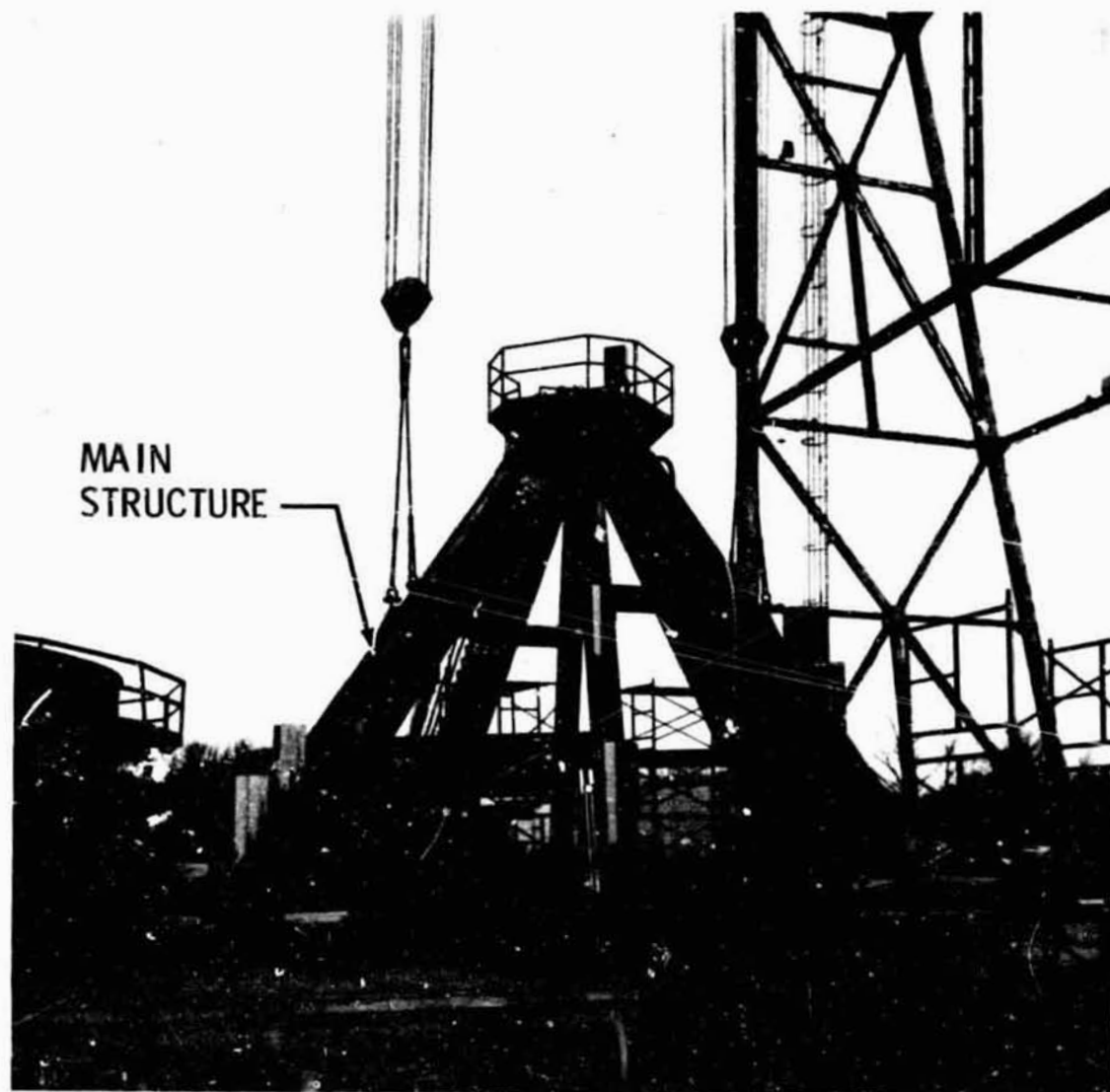
Figure 2. Thrust-Measuring System, Main Structure Pre-Installation
